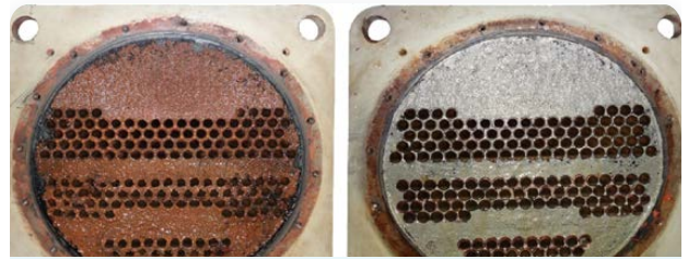
CONDENSER TUBE-SHEET — BEFORE VS. AFTER JC 9450
